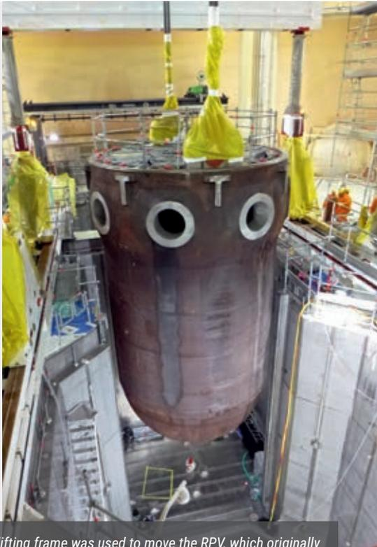
The Mammoet lifting frame was used to move the RPV, which originally weighed 530 t, onto the dismantling frame for the calotte.
