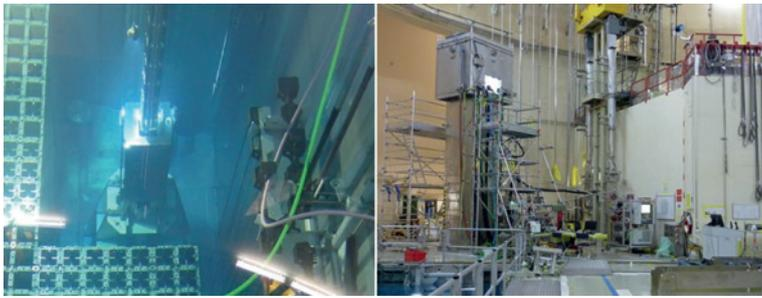
**Fig. 15.** Shielding basket and loading station in the spent fuel pool (left) and the service station with mobile hot cell positioned on the shielding block and equipment on the reactor floor (right).
