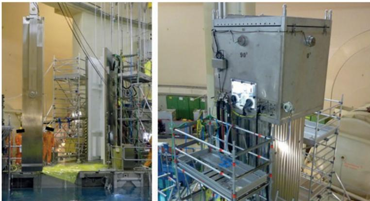
**Fig. 17.** Transport of the shielding basket to the shielding block (left), mobile hot cell (right).
